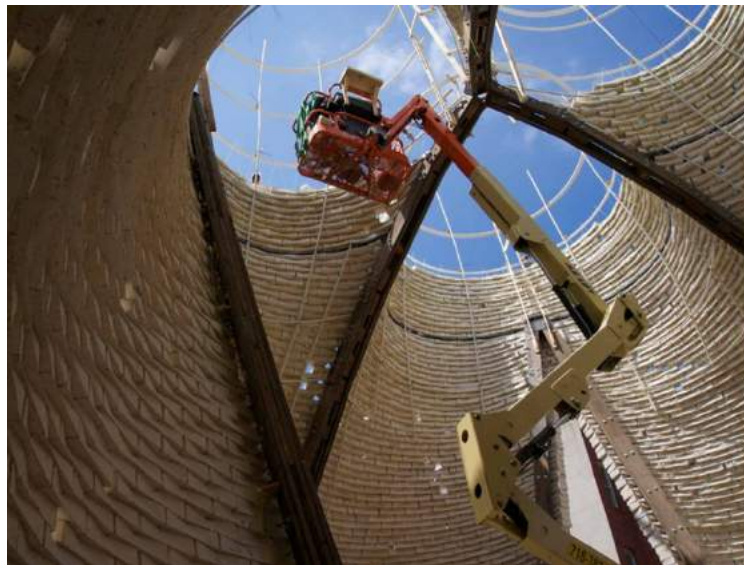
Figure 25. Hy-Fi pavilion is constructed with low energy mycellium bricks for hosting cultural events, after three months the structure was disassembled and composted.
