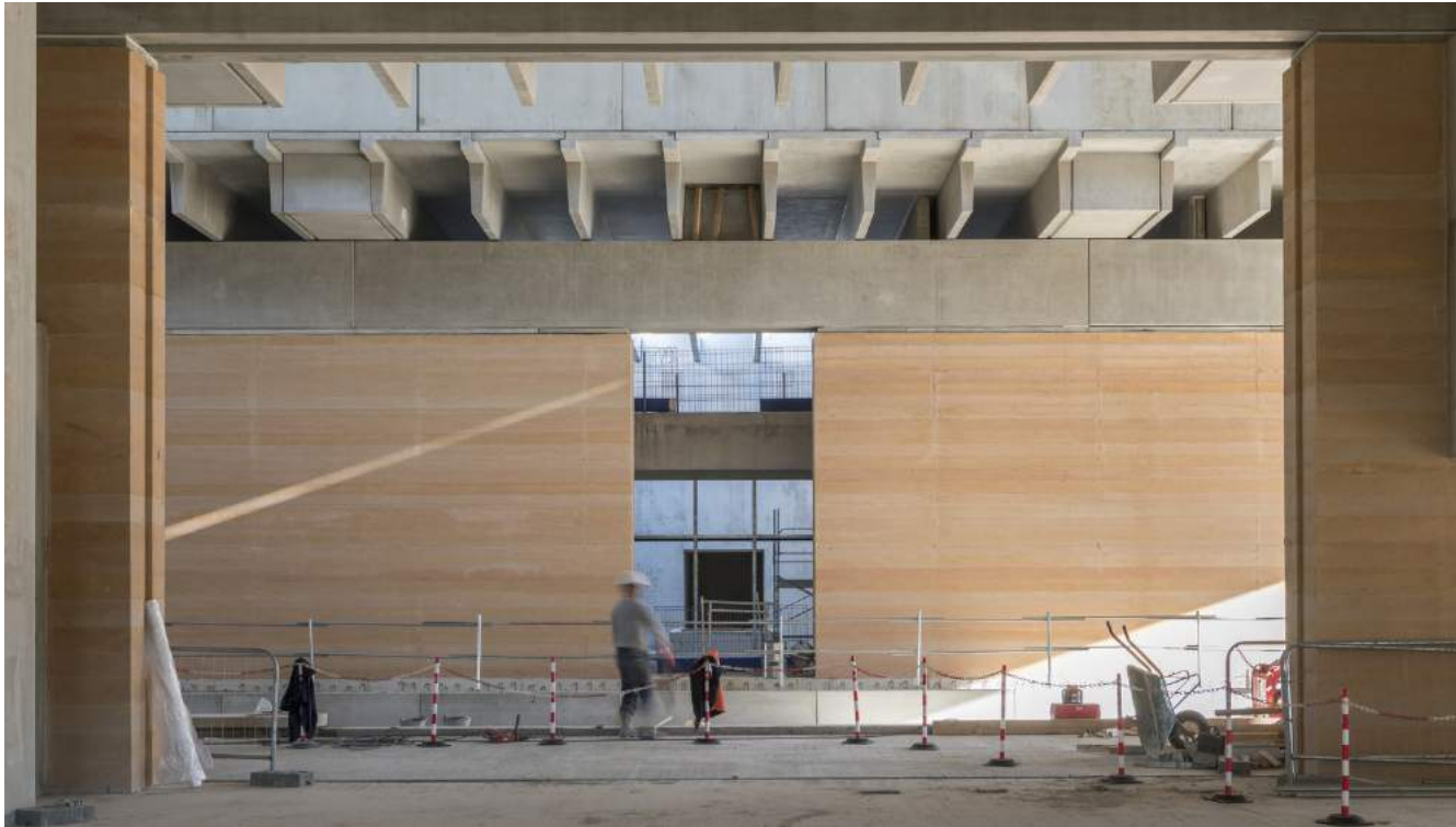
Figure 16. The walls of the Musée Régional de la Narbonne Antique in France, appear to be the environmentally sensitive material of rammed earth but are in fact, a steel-reinforced earth composite with just slightly less cement than a concrete wall.
