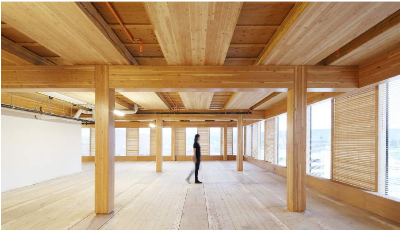
Figure 39. The Wood Innovation Design Centre features an innovative timber post-and-beam structure.
